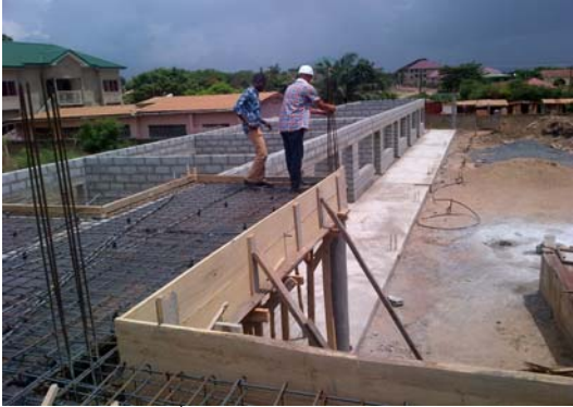
Rebar work on 1 st Floor ceiling of the school
