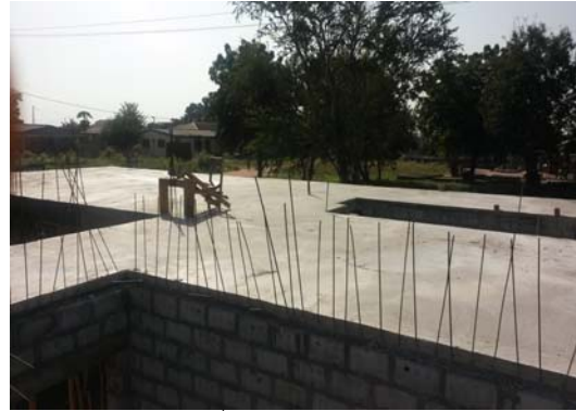
Concrete work on 1 st floor ceiling of school building
