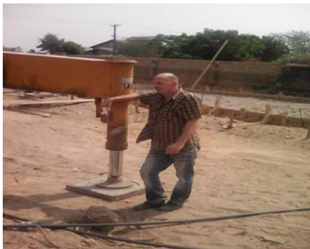
Progress work on New School building
